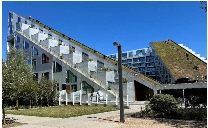
Figura 18. 8 House, Bjarke Ingels Group
